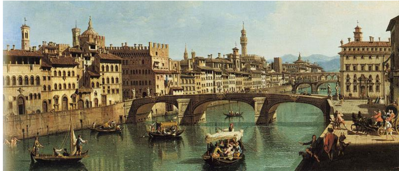
Santa Trinita Bridge, by Bartolomeo Ammannati (1511-1592). Drawing by Giuseppe Zocchi (1711-1767). The vault profiles were designed to minimize the stresses due to bending, drawing inspiration from the natural shape of a hanging wire.
