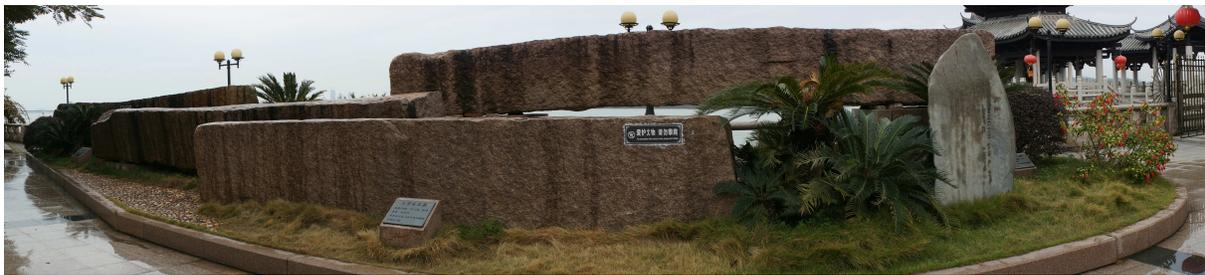
**Fig. 4.** Ancient granite stone beams of the Guangji bridge (number 12), preserved in a park near the bridge. The spans range between 10 and 14 m.
