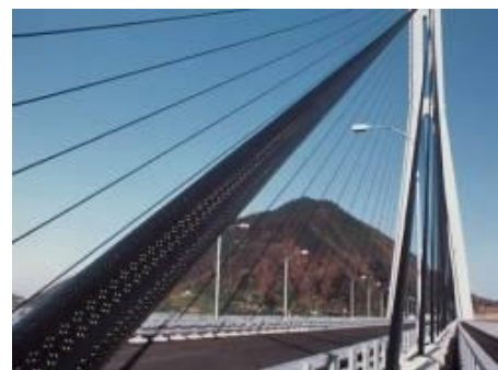
(a) Helical wire (Akashi Kaikyo) (b) Additional damping (Kurushima Kaikyo) (c) Cross tie & Rigid tie (Hitsuishijima / Iwakurojima) (d) Indent cable (Tatara)
