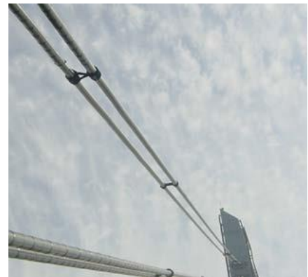
Figure 13: Alternative countermeasures by rigid tie with damper
